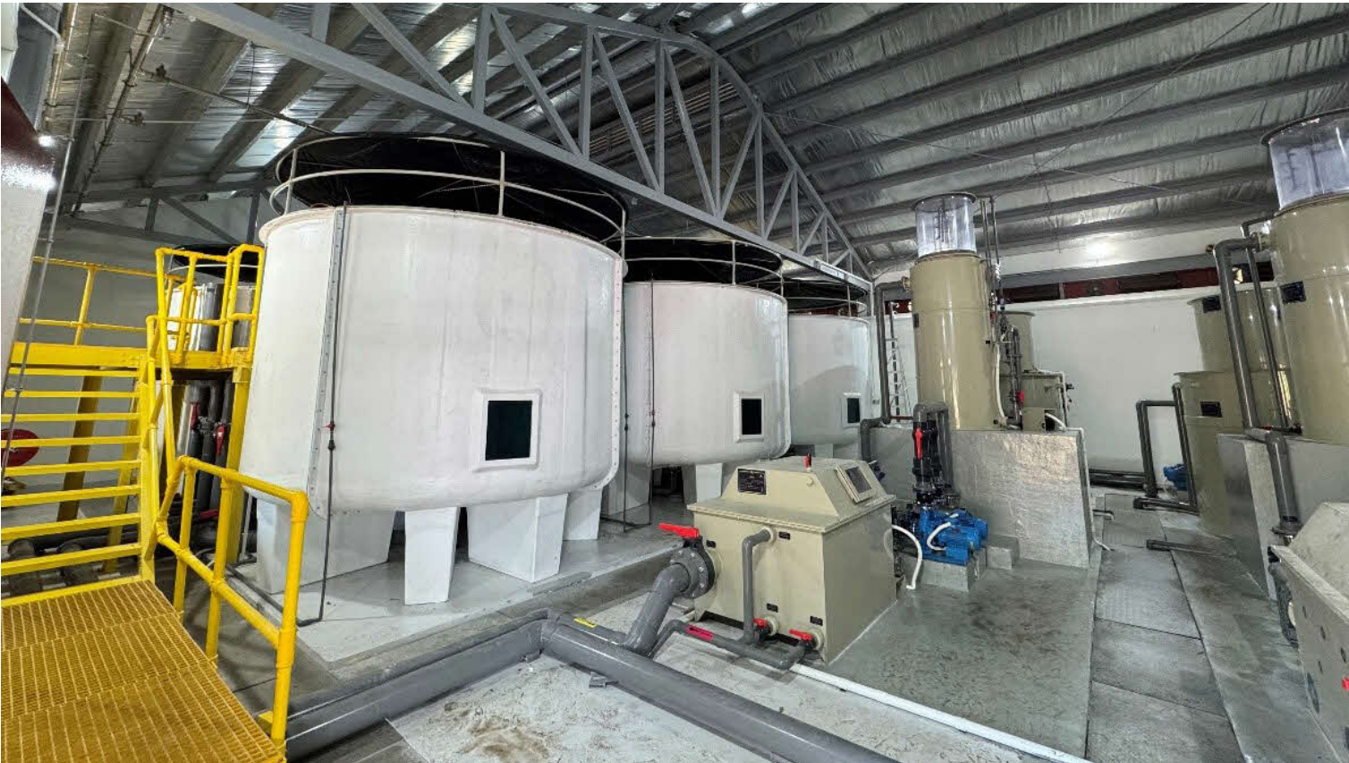
▲ SFA's Marine Aquaculture Centre's indoor broodstock facility is equipped to operate either as a fully recirculating system or as a flow-through system for Asian seabass brooders.
