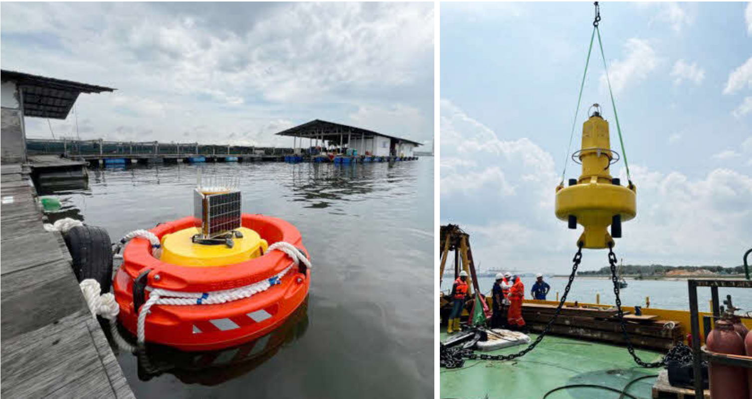
▲ Deploying and installing ASN real-time monitoring stations.
