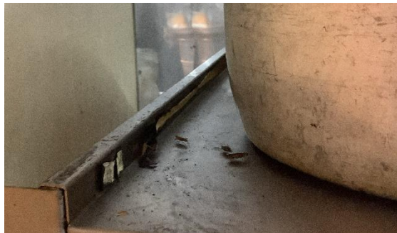
Cockroach Infestation at food preparation areas (Photo by SFA)
