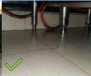
Clean floor under cabinet
