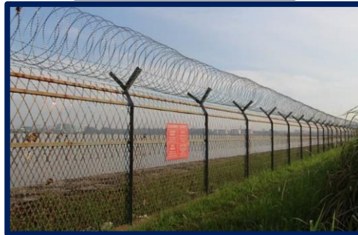
Fencing at Punggol Barat
