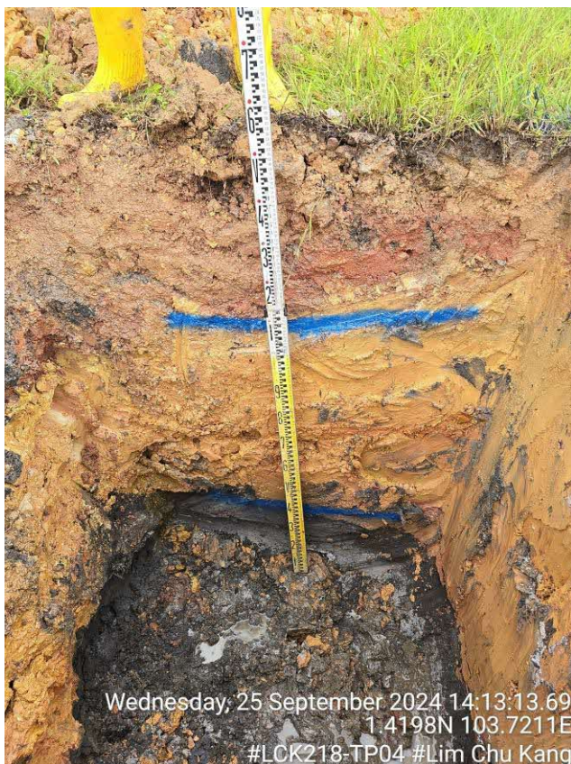
Figure 3.16 Closeup View of Trial Pit LCK218-TP04
