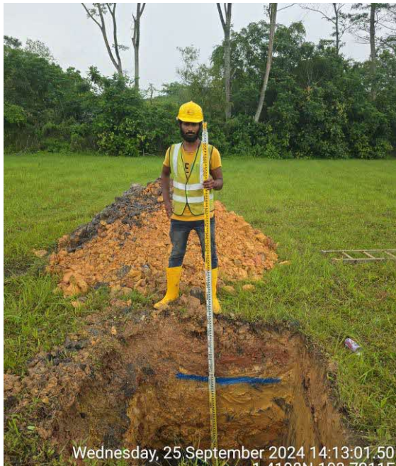
Figure 3.15 General View of Trial Pit LCK218-TP04
