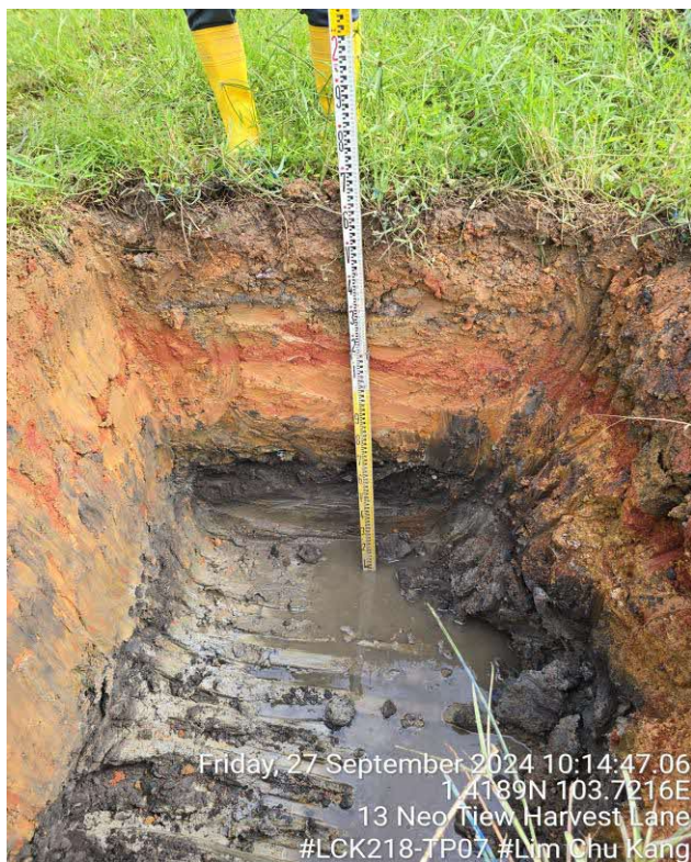
Figure 3.28 Closeup View of Trial Pit LCK218-TP07
