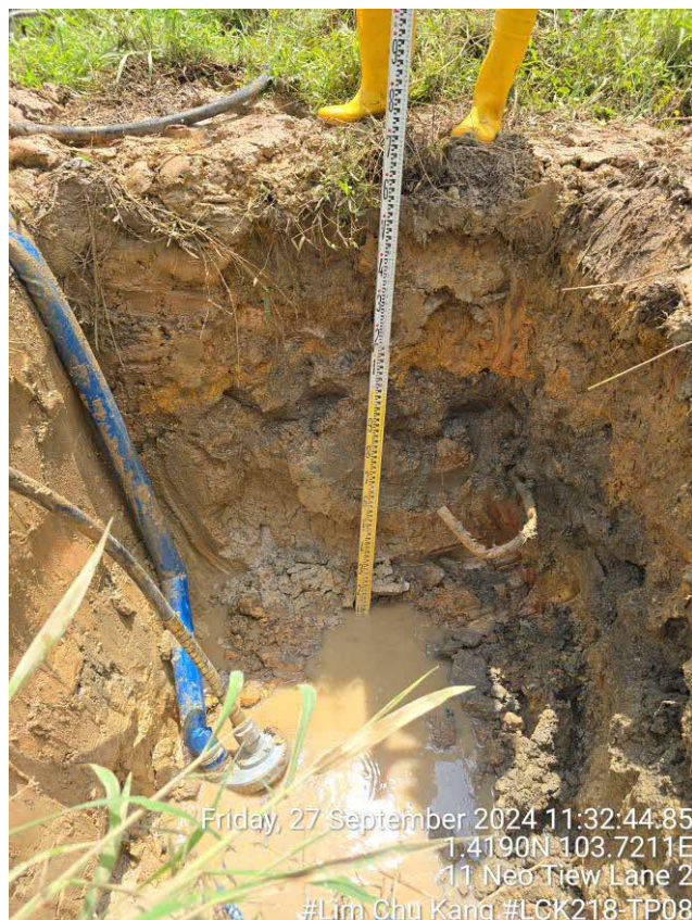
Figure 3.32 Closeup View of Trial Pit LCK218-TP08
