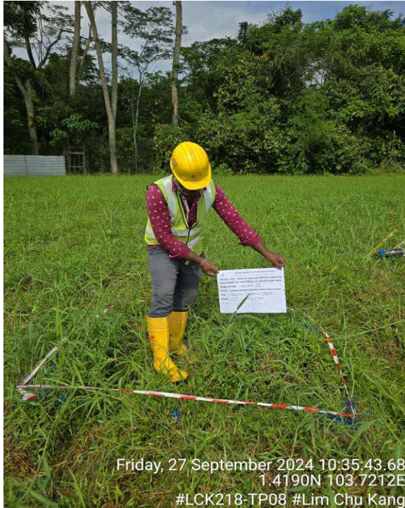
Figure 3.29 Trial Pit Location for LCK218-TP08
