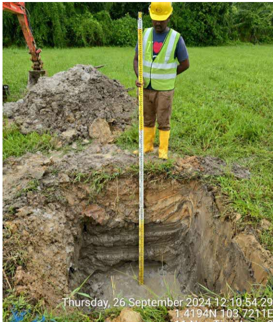
Figure 3.19 General View of Trial Pit LCK218-TP05
