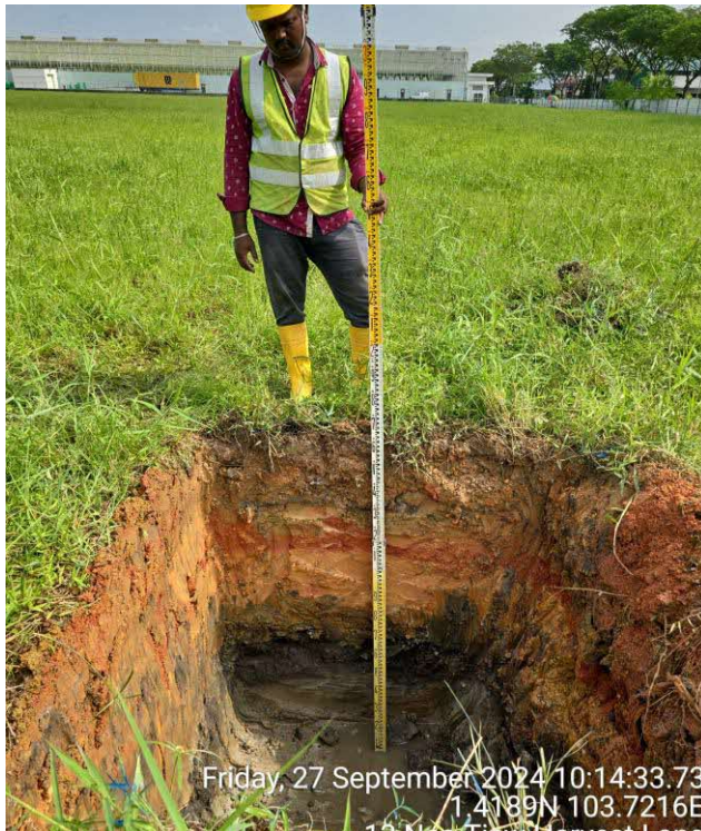
Figure 3.27 General View of Trial Pit LCK218-TP07
