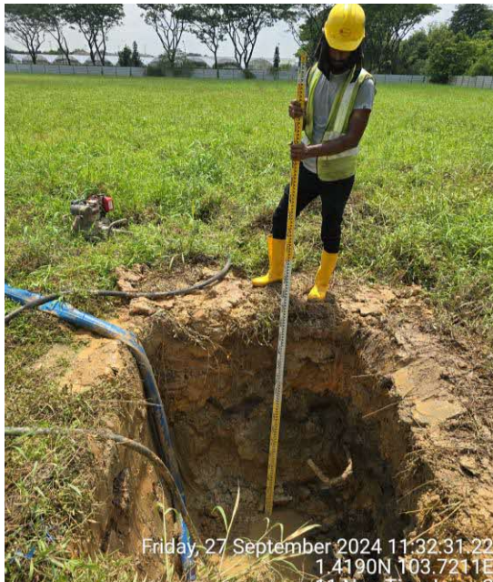
Figure 3.31 General View of Trial Pit LCK218-TP08
