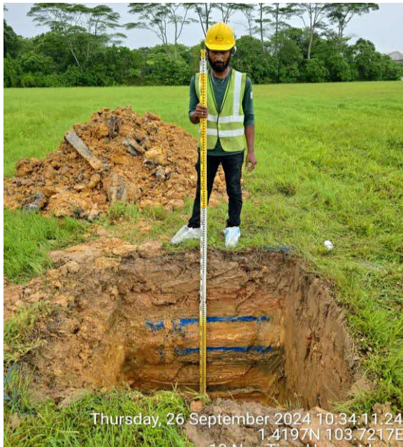
Figure 3.11 General View of Trial Pit LCK218-TP03
