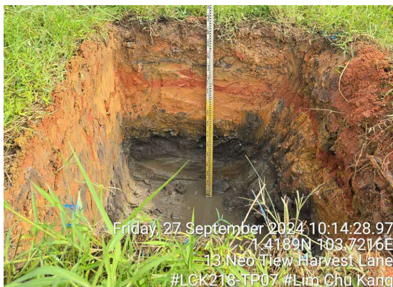
Figure 3.26 Overview of Trial Pit LCK218-TP07
