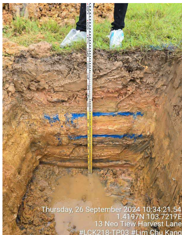
Figure 3.12 Closeup View of Trial Pit LCK218-TP03
