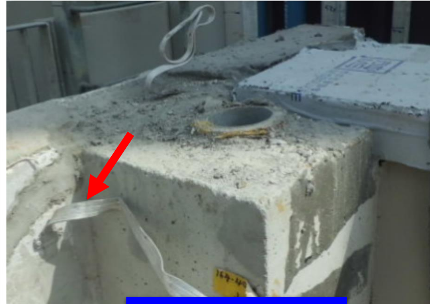
Incomplete lightning conductor
