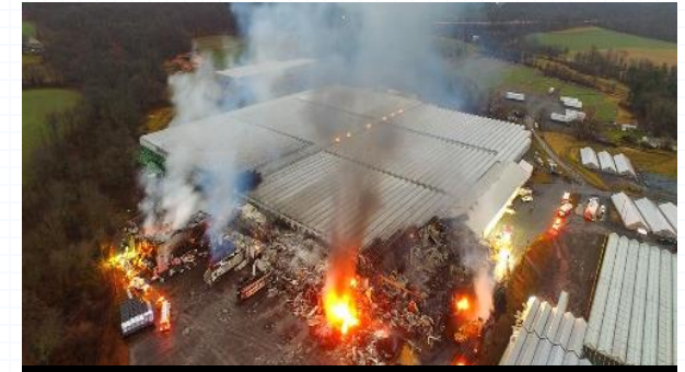
In 2017, Greenhouse fire in Pennsylvania, USA. The roof of the building collapse.
