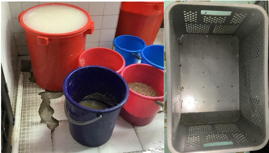
Left: Poor maintenance (broken floor tiles) within the premises
